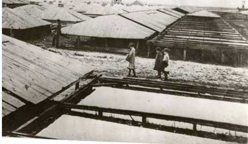
Figure 28: West Yarmouth Salt Works Source: https://newenglandhistoricalsociety.com/the-rise-and-fall-of-cape-cod-salt/
